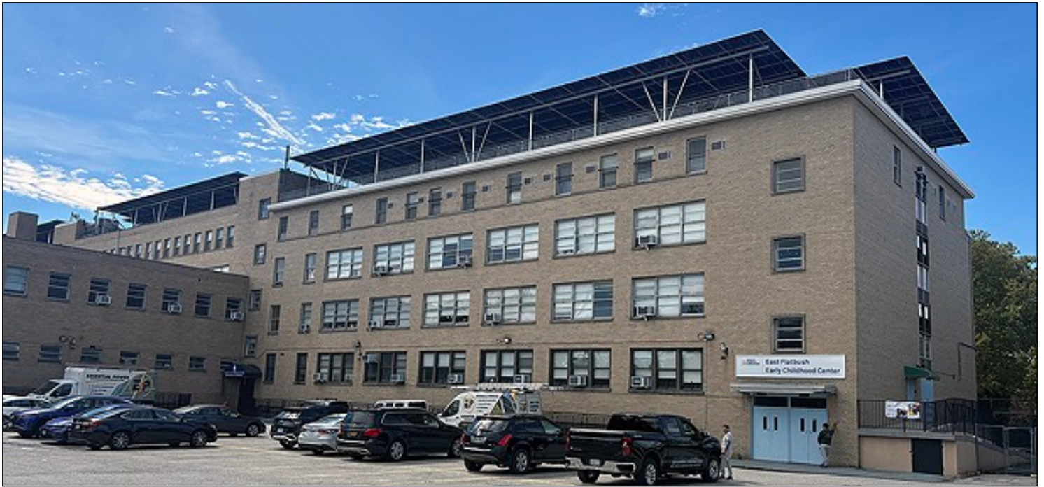
Panels seen from the parking lot (the track, for old-timers). They run along the main part of the building, but not above the gym.
