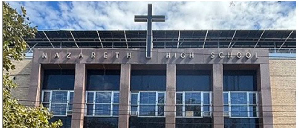
Above, a view over the front entrance of the school on 57th Street; below, equipment on the way to being installed in the basement.
